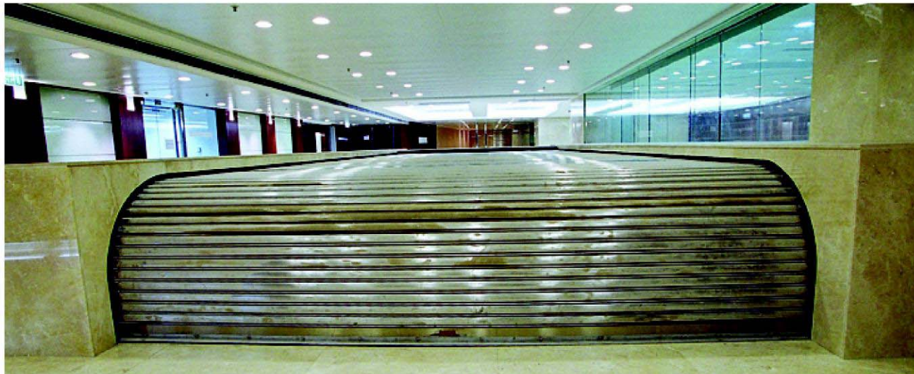
The fire rated horizontally sliding shutter is for escalator fire protection.
